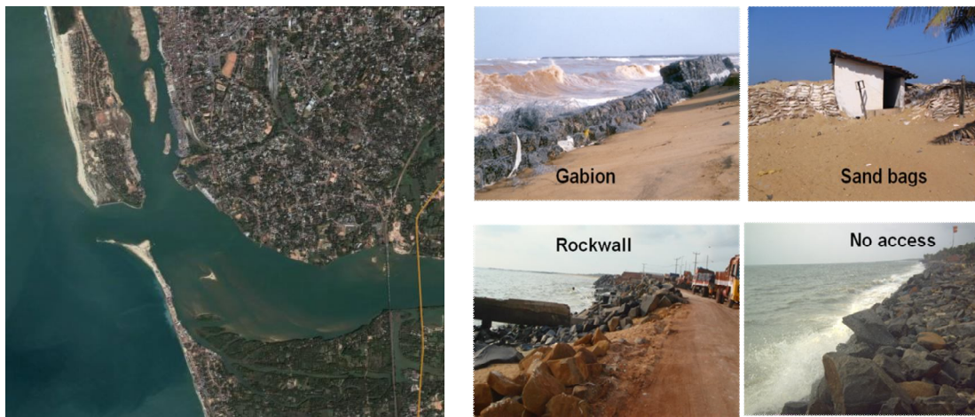
Figure 27: Location of Mangalore Inlet and status of erosion and temporary protection work being carried out every monsoon since past one decade
