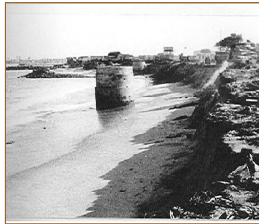
A View of erosion north of Chennai Harbour Break water is seen in back ground (June 1978)
