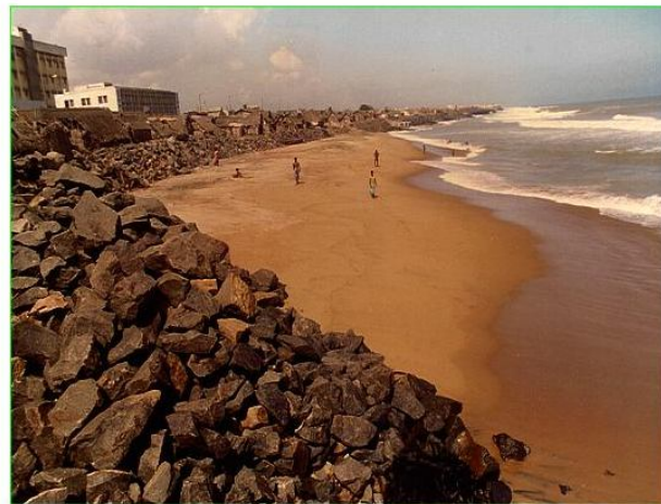
Fig. 14 - Sea wall along Rayapuram
