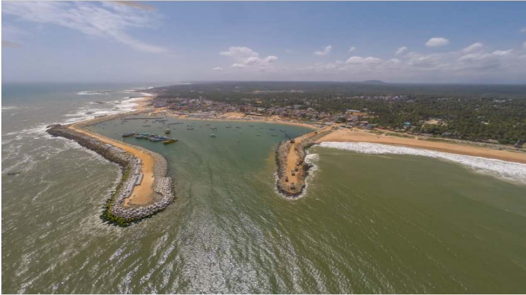
Colachel Fishing Harbour ongoing work at a cost of Rs 87.75 crore
