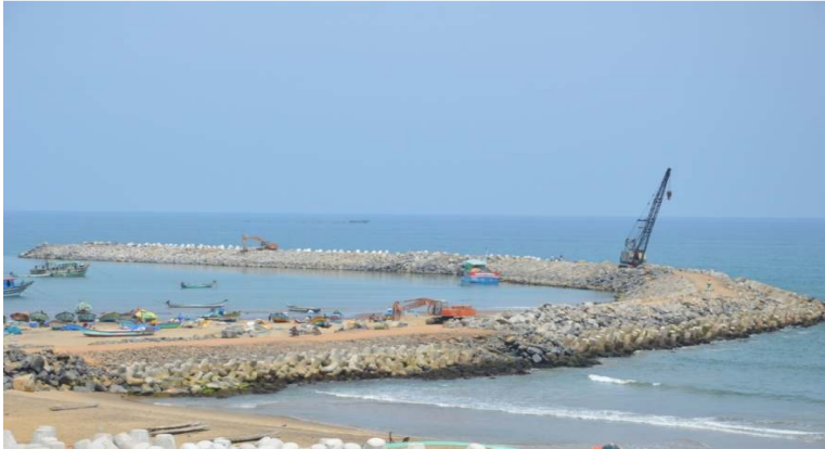
Poompuhar Fishing Harbour ongoing work at a cost of Rs 148 crore
