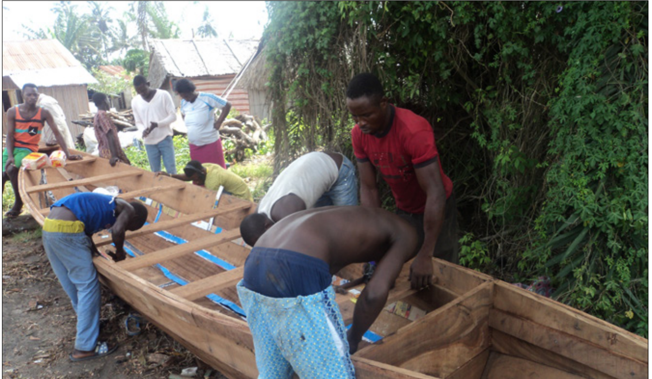
Construction of a planked canoe at Ikosi-Agbowa fishing community, Lagos. Small-scale fishers and fish processors continue to operate during the pandemic but their incomes and profits have declined because of the loss of customers.
