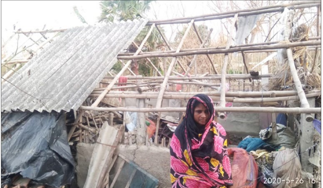
Impact of Amphan cyclone, south 24 Parganas, India. The devastation of cyclone Amphan was wide-ranging. Besides shattering the livelihoods of communities, the cyclone destroyed basic amenities like shelter, housing, food, healthcare and education
